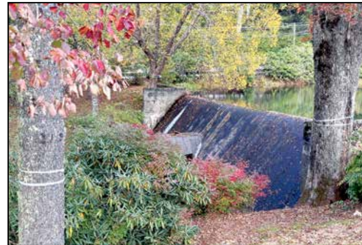
Spill dam at Highlands Country Club.
