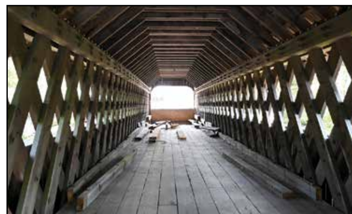
The bridge was reconstructed, retaining the lattice style design that was patented by Ithiel Town in 1820 and 1835. Graton's reconstruction process was meticulous, using centuries-old craft techniques and replacing rotten, insect-ridden, or unstable parts.
