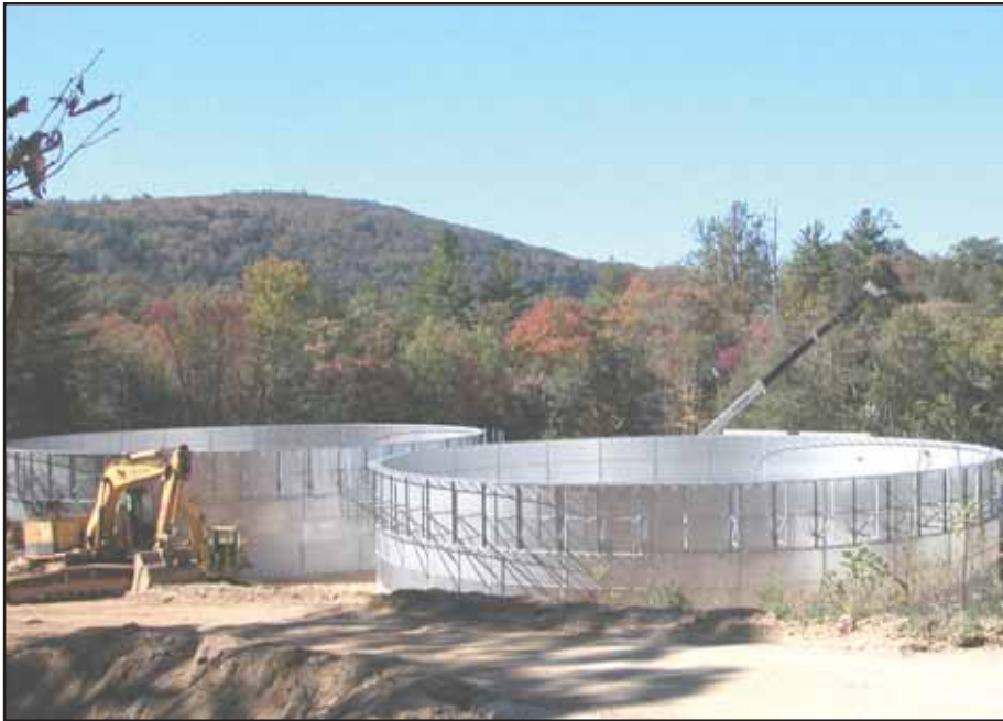
New stainless steel processing tanks are being added as part of the $5.9 million expansion project from 50,000 gallons a day capacity to 150,000 gallons a day capacity. Photos by Jim Lewicki
