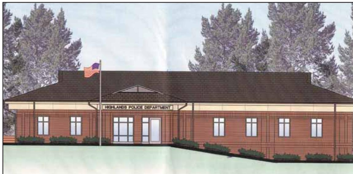
A trussed roof would be added to the structure that previously housed the Highlands ABC Store and brick veneer broken up visually with contrasting brick or rock will be attached to the exterior.
